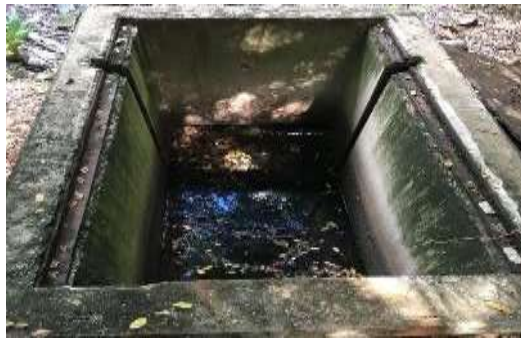
Figures 3.10 & 3.11: – Inner Drainage Overflow Structure (3.11) and Outer Drainage Overflow Structure (3.12) – School site.
