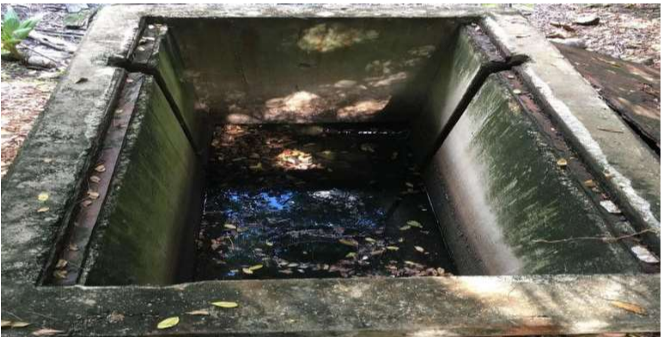
Inner Drainage Overflow Structure
